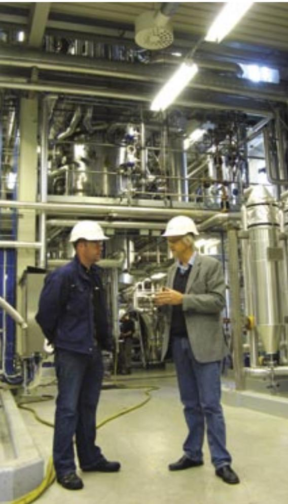
The BLEF-DME is designed as an integral part of a pulp mill substituting a recovery boiler. The efficiency is high due to a shift to more advanced technology in the chemical recovery unit of the pulp mill.
